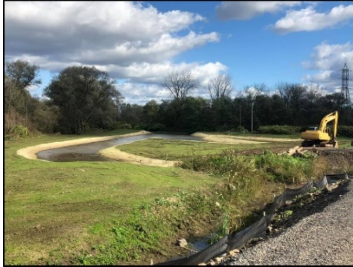
Figure 5: Project 2 – Return floodplain bench, Whitesboro, NY.
