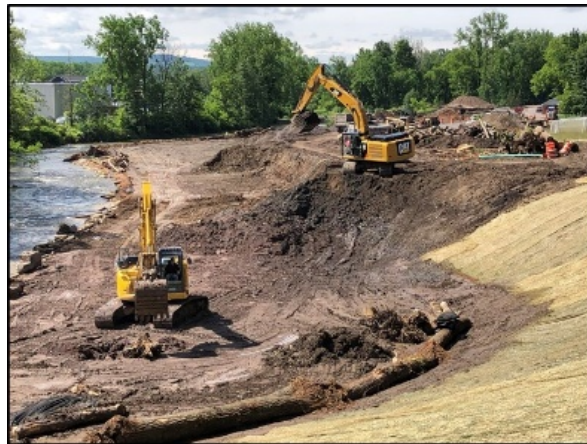
Figure 3: Construction of Project 1.
