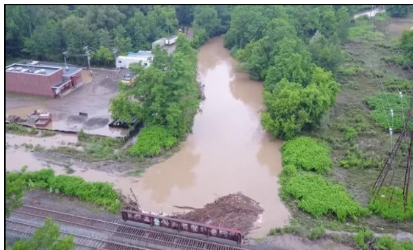
Figure 2: Flooding at the CSX Bridge: 2019 Halloween Storm - Whitesboro, NY
