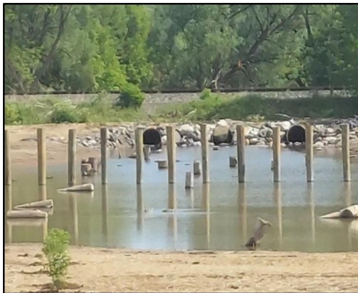
Figure 6: Project 2 – Culverts and floodplain bench, Whitesboro, NY.
